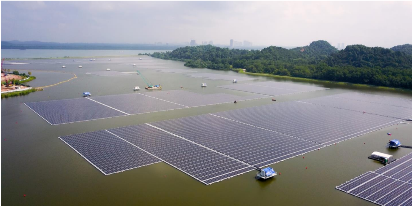
Currently under construction
