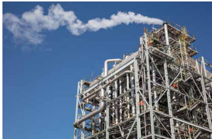
Sembcorp Cogeneration Plant, Sakra on Jurong Island, Singapore
