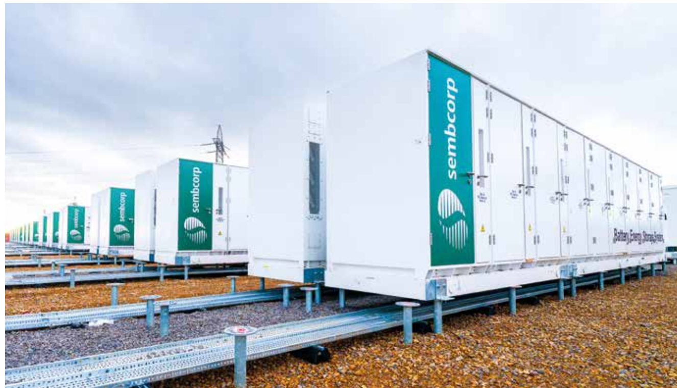
Battery energy storage system under construction at the Wilton International site on Teesside, UK
