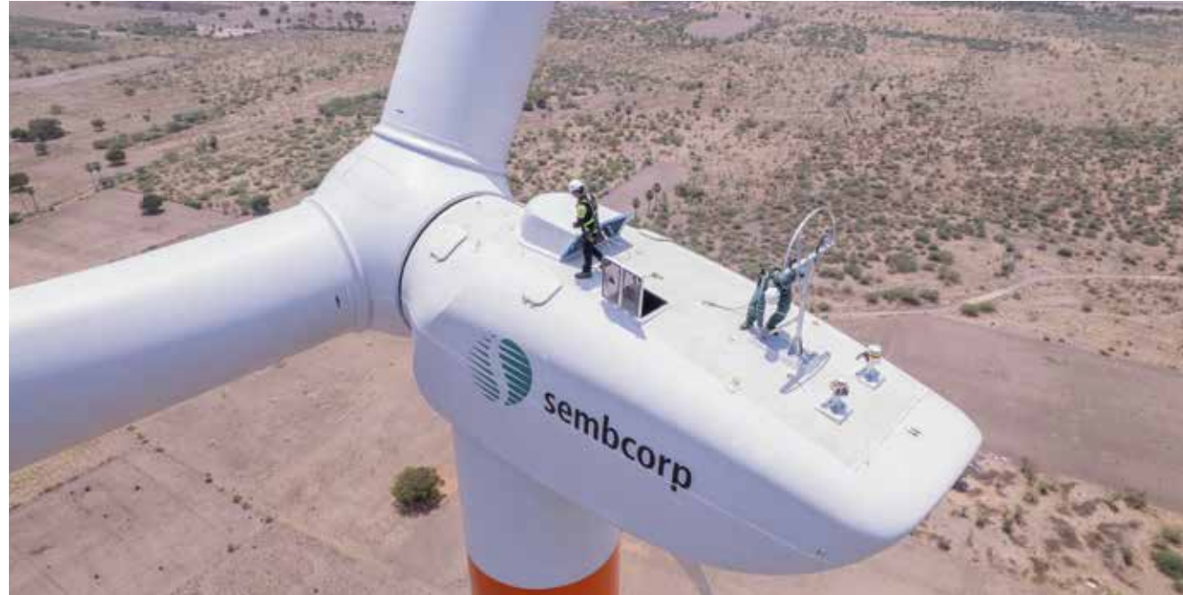
Conducting maintenance on a wind turbine in India
