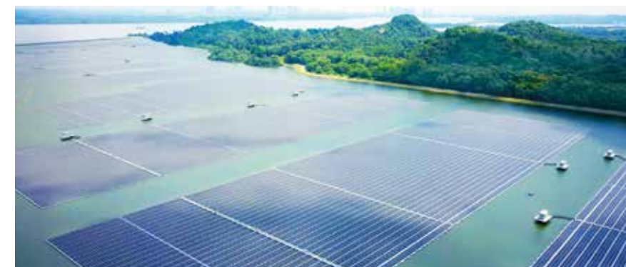
Sembcorp Tengoh Floating Solar Farm in Singapore
