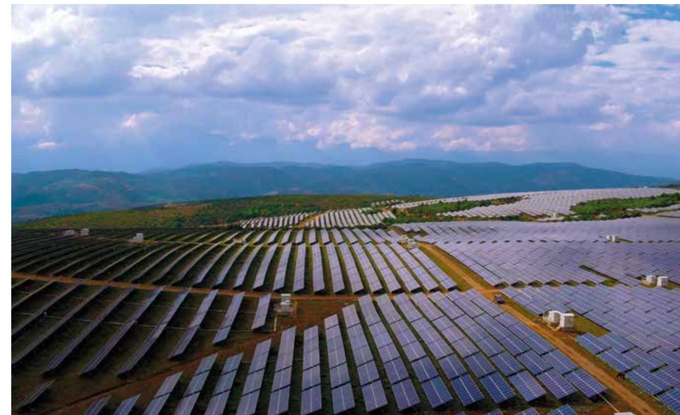
Sembcorp solar assets in Yunnan, China
