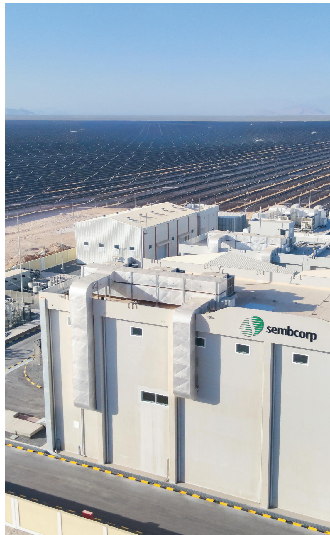
Sembcorp's Manah II Solar Independent Power Project in Manah, Sultanate of Oman
