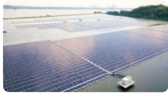
Sembcorp Tengah Floating Solar Farm
