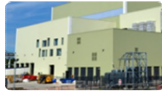
Sembcorp biomass plant
