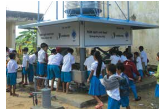
→ Building water systems to deliver clean water to 14,000 people in rural Vietnam.
