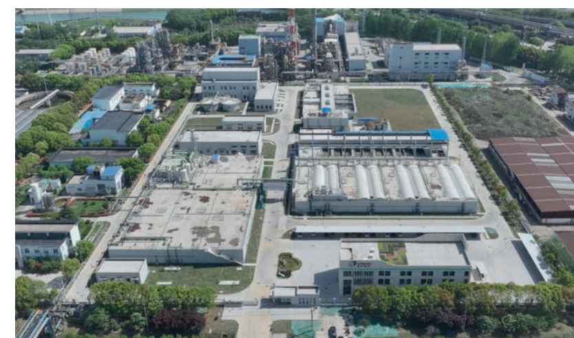
Sembcorp Nanjing Suiwu Wastewater Treatment Plant, China
